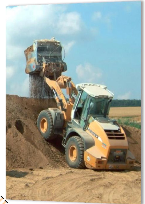
SkanCraft conditioner & lime dosing unit preparing soil
