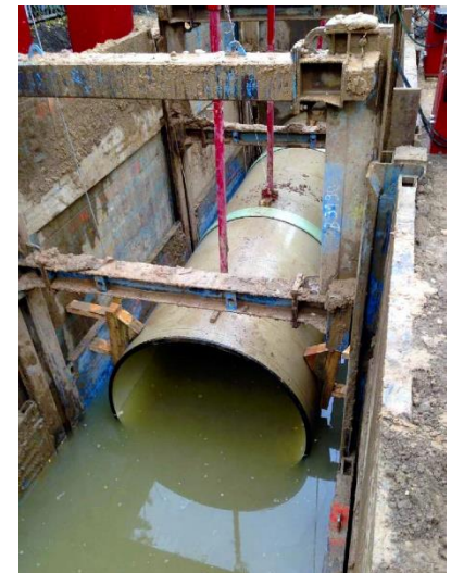
Pipe laying in groundwater with RSS Flüssigboden®
