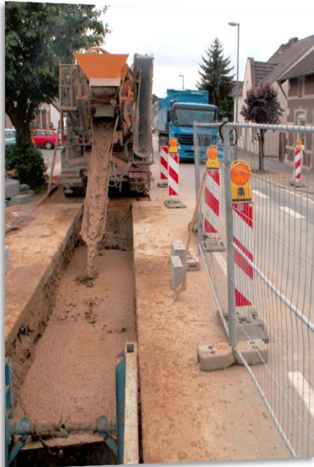
Refilling of trench
