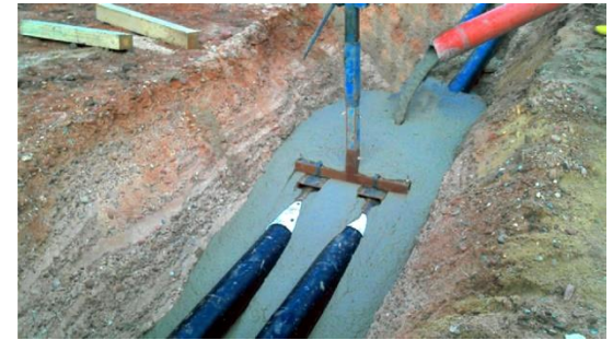
District heating lines embedded in RSS Flüssigboden®
