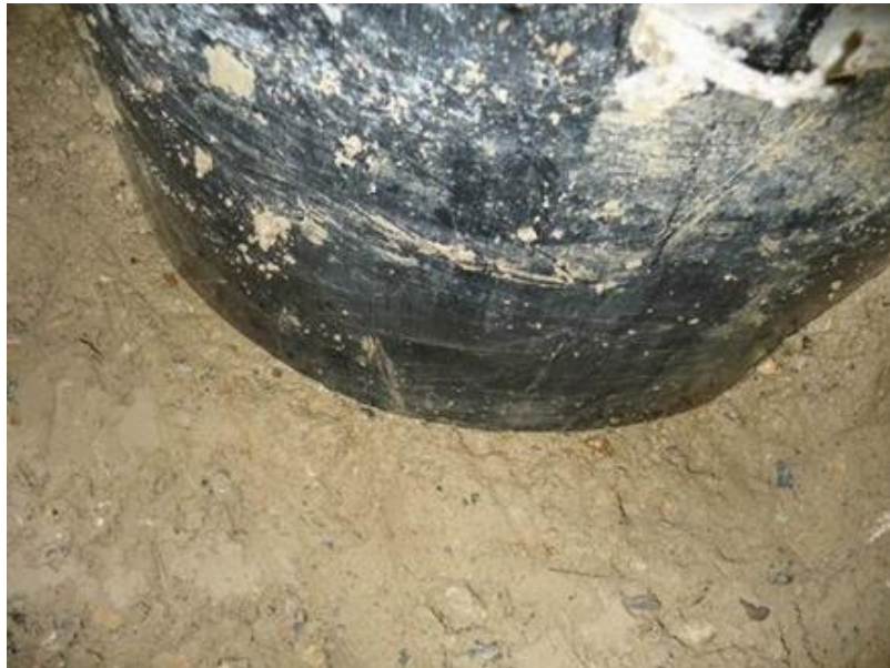
Source: Archive RSS Flüssigboden® building sites
