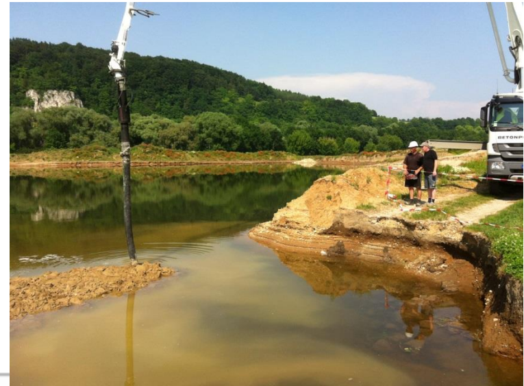
Source: Archive RSS Flüssigboden® building sites
