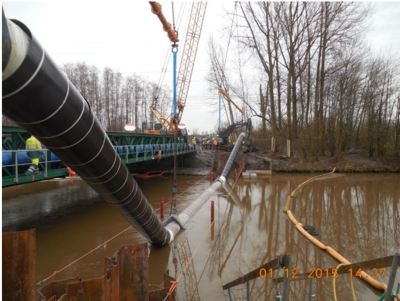
Source: Archive RSS Flüssigboden® building sites
