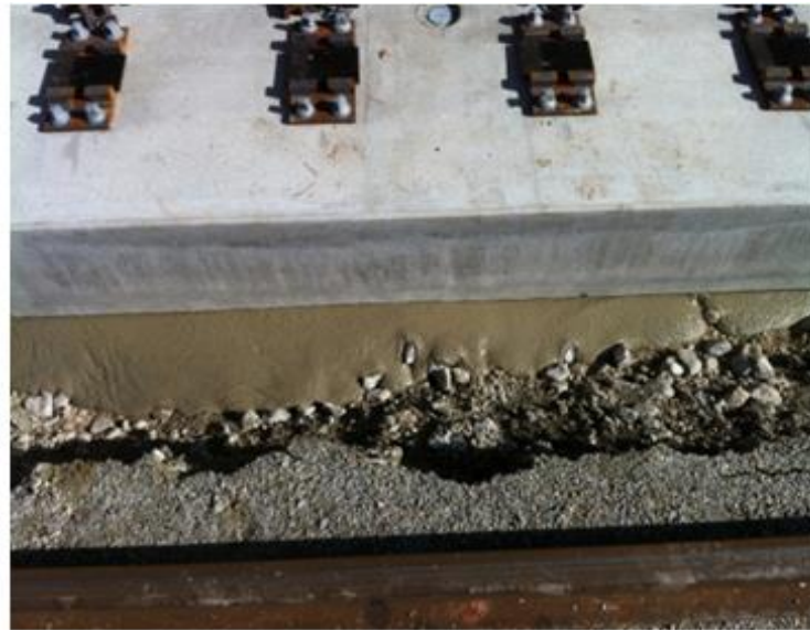
Source: Archive RSS Flüssigboden® building sites
