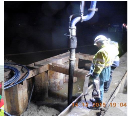
Source: Archive RSS Flüssigboden® building sites
