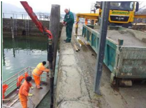
Source: Archive RSS Flüssigboden® building sites
