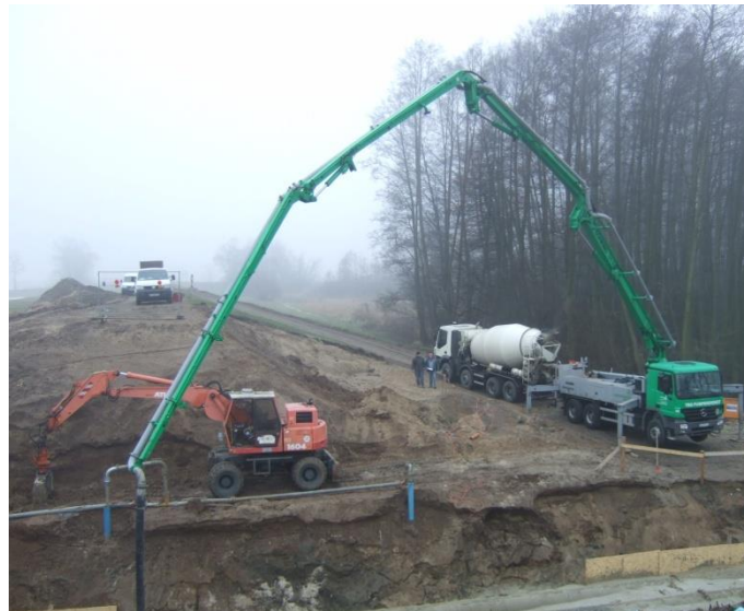
Source: Archive RSS Flüssigboden® building sites
