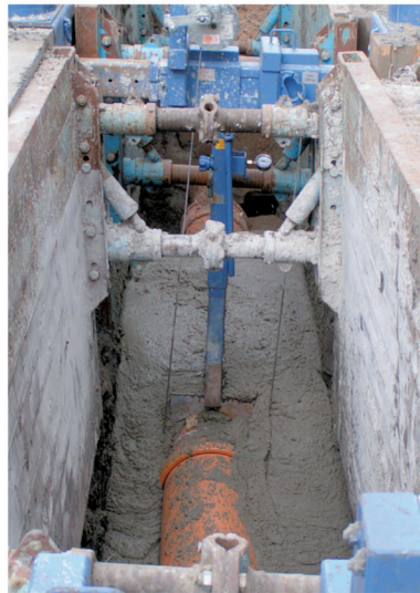
Floating pipe laying
