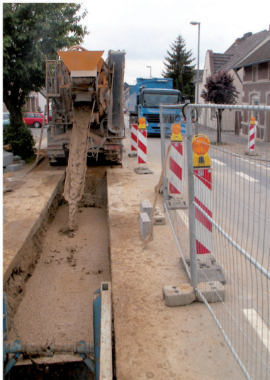
No compaction required – narrow construction sites with no full closures required
