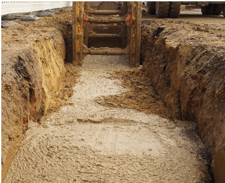
Trench backfilled with RSS® Flüssigboden
