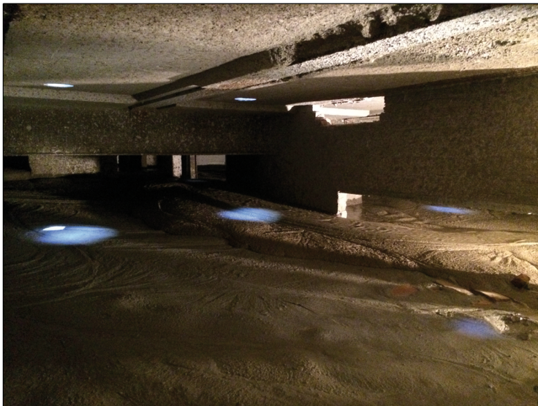
Subway tunnel Dresdner Straße backfilling
