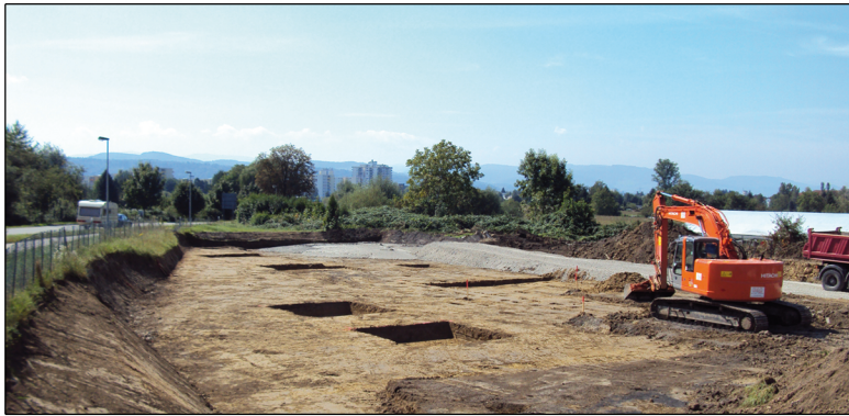
Technology of a foundation slab with RSS® Flüssigboden
