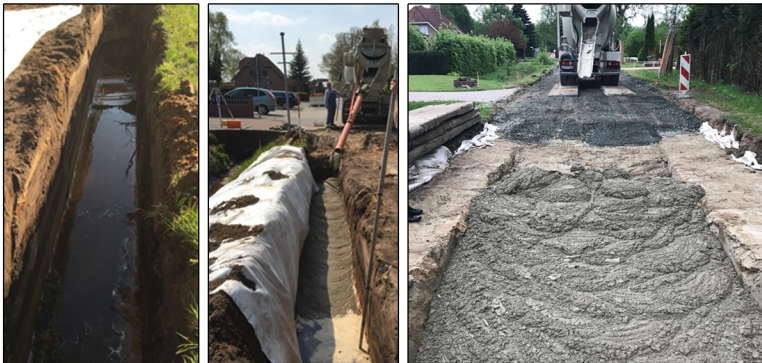
Technology of a framed foundation slab with RSS® Flüssigboden
