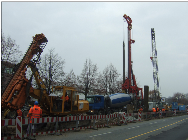
Backfilling of drilled piles with RSS® Flüssigboden
