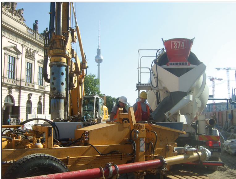
Backfilling of drilled piles with RSS® Flüssigboden
